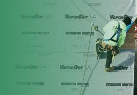
A unique self-adhered roofing membrane with vapor permeability, reducing potential of damage due to moisture build-up
