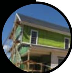
Slicker® Classic is the original rolled rainscreen. The unique, vertically-channeled, three-dimensional matrix of Slicker provides a continuous space for drainage and drying—eliminating the threat of trapped moisture.
