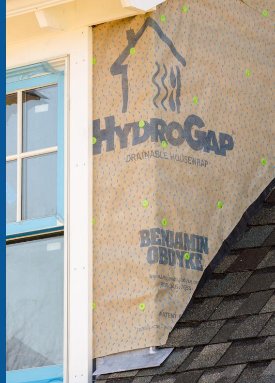
*[HydroGap] gave us a house wrap that will protect the framing and an effective drainage plan, is also robust enough that it can withstand the high winds of a waterfront location before it is covered.*
