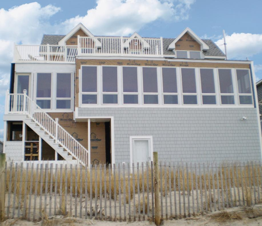
*Because the housewrap used on the home didn't allow the wall structure to breathe, intruding moisture was able to sit in the wall assembly before it finally forced its way into the structural elements, causing rot and mold.*
