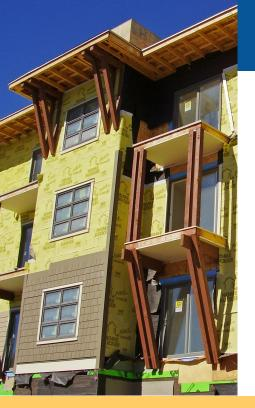
Plus Typar will deliver the combined benefits of a rainscreen and water resistive barrier behind the siding. Each roll contains the patented Slicker three-dimensional matrix bonded to Typar, the premium residential and commercial grade housewrap by Fiberweb Incorporated. This combination allows moisture to drain and dry quickly before it damages sidewall materials and protects the wall assembly from mold and rot.
